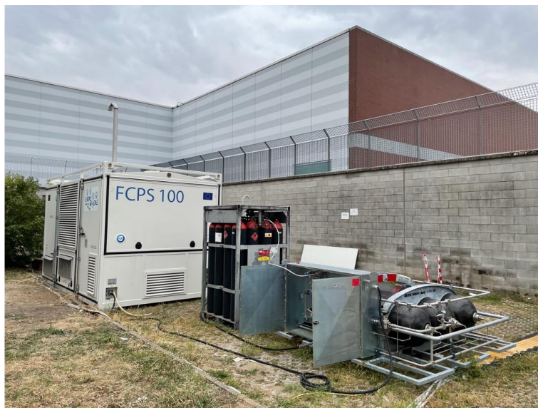
Figure 4 Example of test on site for EVERYWH2ERE Genset with bundles
