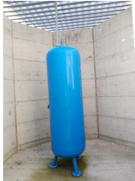
Figure 13 Storage system of gaseous hydrogen and containment structure required (Italy)
