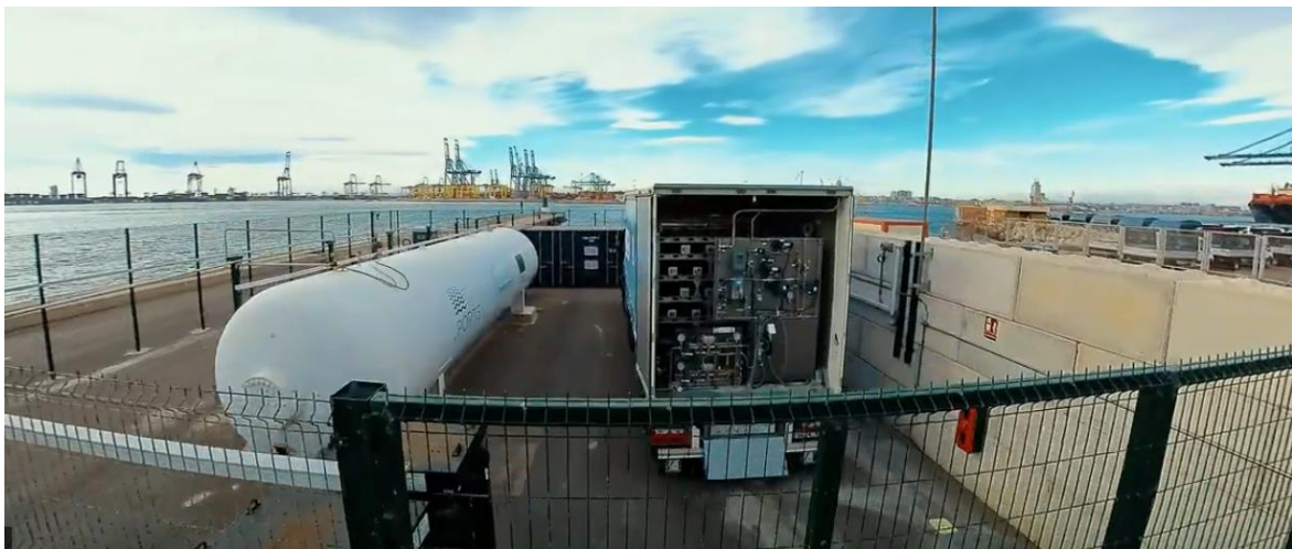
Figure 12 HRS system installed in the Port of Valencia ( courtesy of H 2 Ports)
