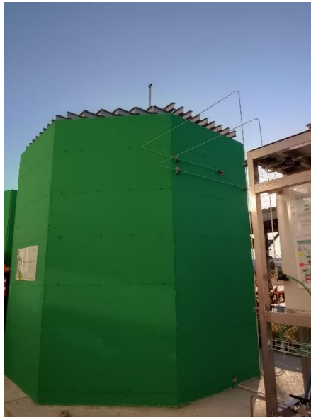
Figure 13 Storage system of gaseous hydrogen and containment structure required (Italy)
