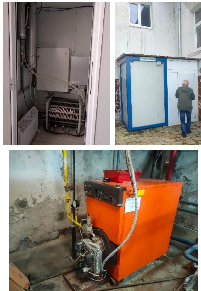
Figure 16 Hydrogen production, containment structure and Heating system for School heating (Bulgaria)
